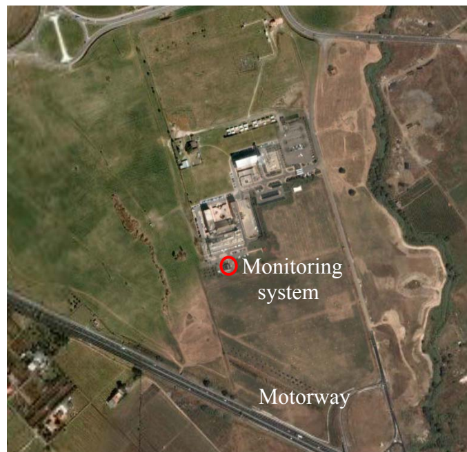
Fig.1. Aerial view of the monitoring system installed at CNR-IA and the nearby motorway.
